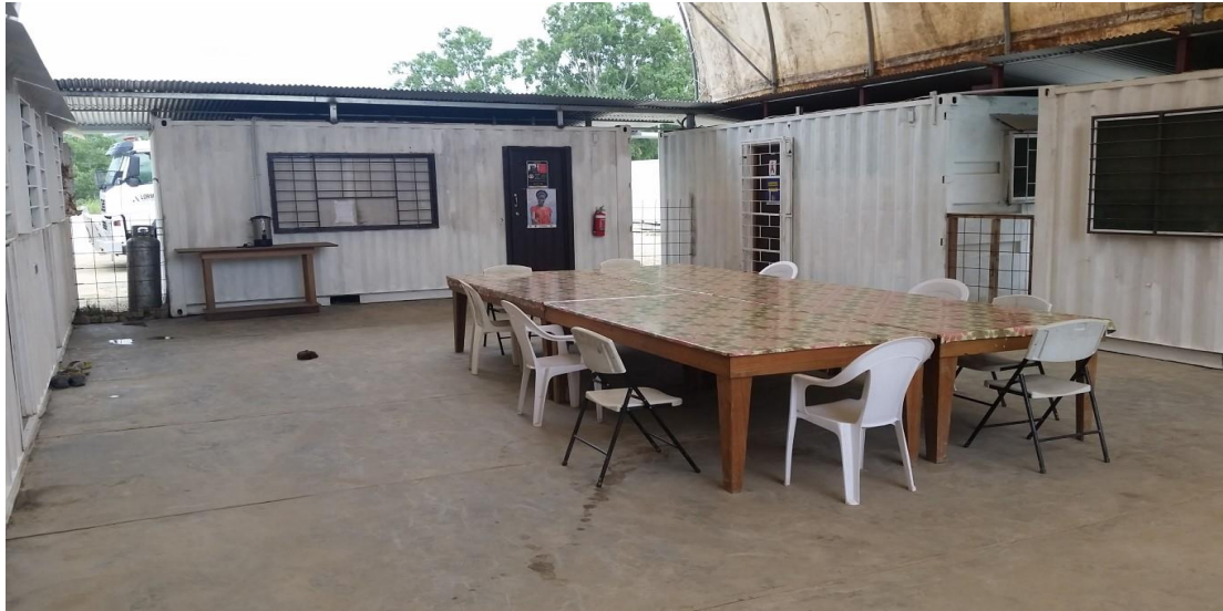
Figure 14: Typical office accommodation inside converted TEU containers
