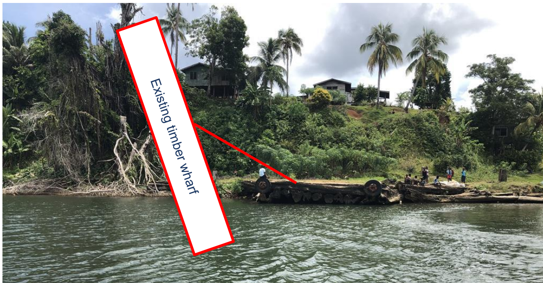
Figure 9: Existing Viru Wharf (March 2019)
