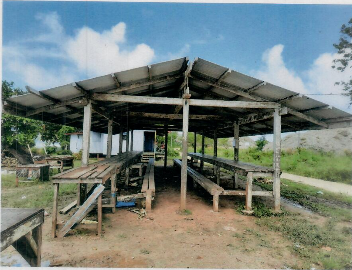
Figure 2: Existing Seghe market-looking south
