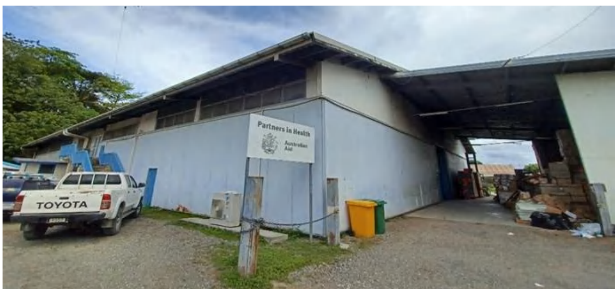
Figure 1.1. Front view of the NMS building
