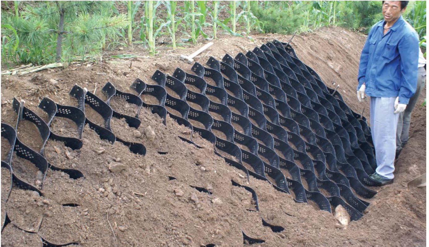
Figure 8: Geotextile matrix used for slope stabilisation (Source: https://www.okorder.com/p/hdpe-geocell-with-certificate-for-road-construction_1031785.html )
