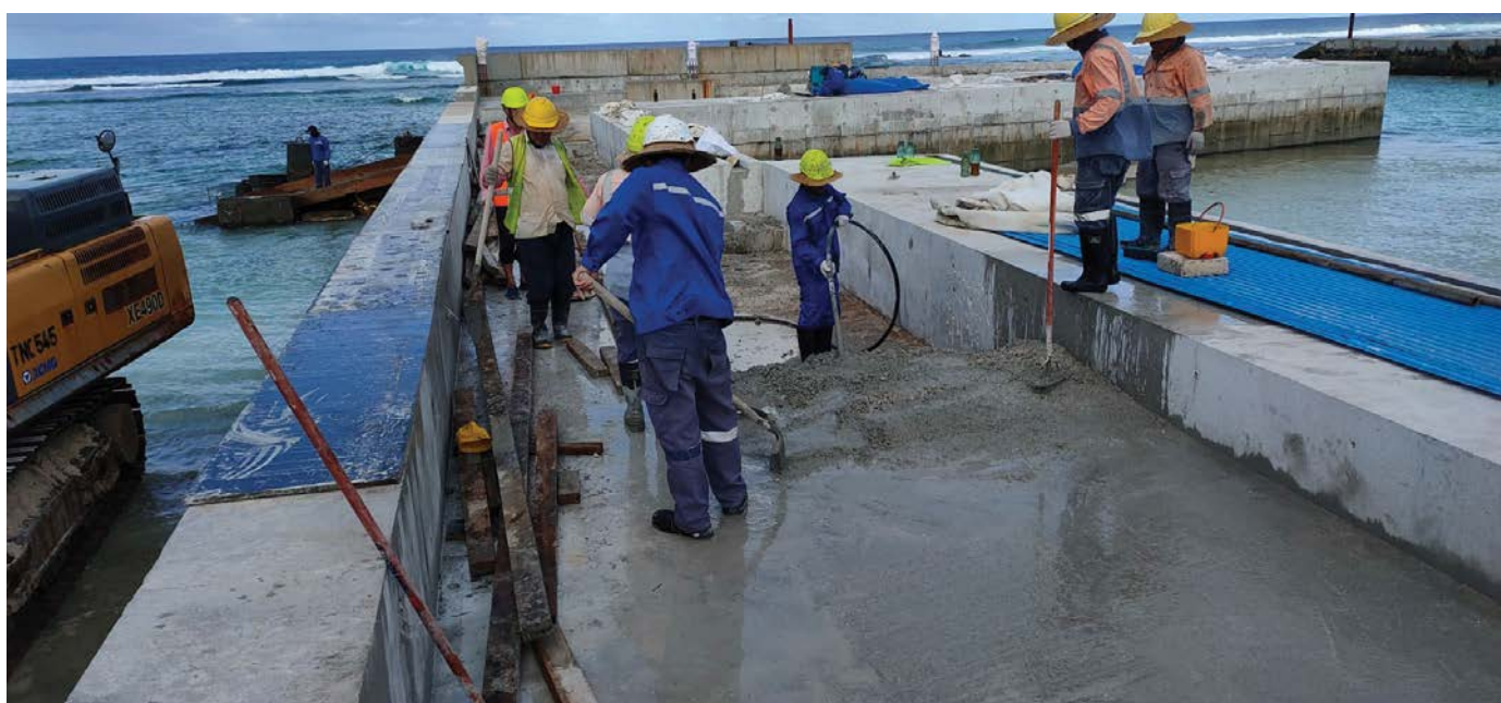
Figure 12: Example of working in low tide conditions and bunding in Nukulaelae, Tuvalu
