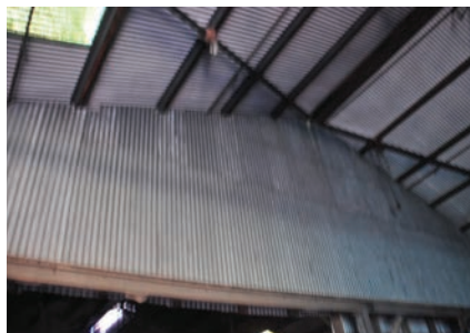
Asbestos wall panels
