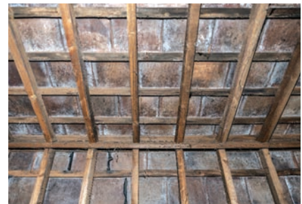
Under the roof
