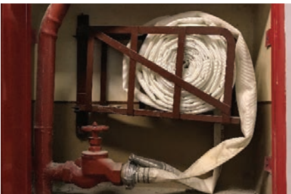
Backing board of fire extinguisher box
