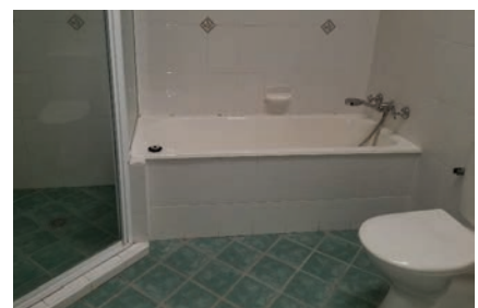
Walls and sink area of bathroom (wet area)
