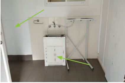
Walls and sink area of laundry (wet area)
