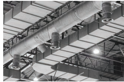
Gaskets on pipe joints
