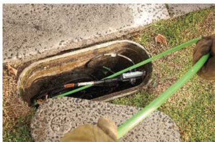
Inside telecommunication pits or other service pits
