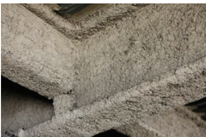
Sprayed insulation under the roof
