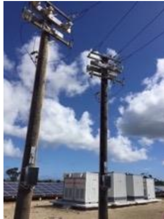
Plate 3.1a: Invertors, transformer and Power lines at Vaini Solar Plant
