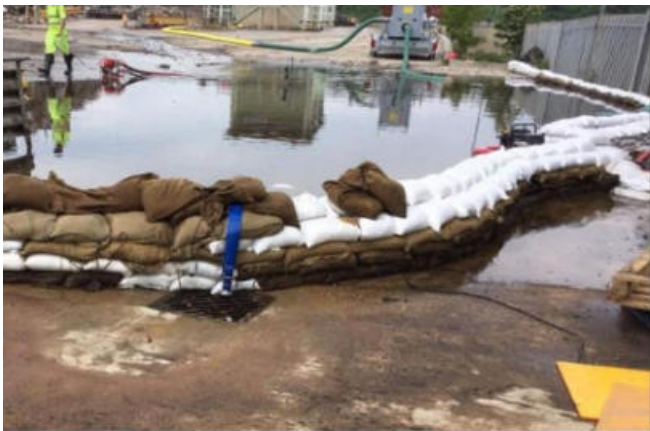
Plates 5.3 a and b: Typical settlement pond and spill boom
