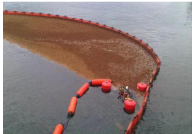
Plates 5.3 a and b: Typical settlement pond and spill boom
