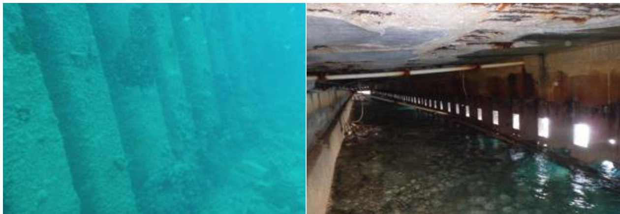
Plates 4.3 a and b: Sheet piles (a) seaward and (b) shoreward of Wharf 1
