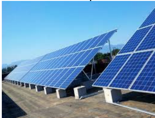
Figure 3.5: ‘Solid state’ silicon solar panels with ballast foundations
