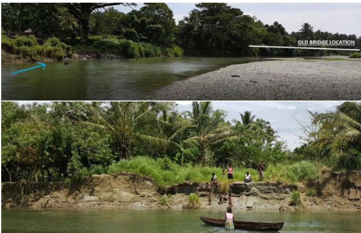
Figure 5: View across proposed Location showing highly erodible banks
