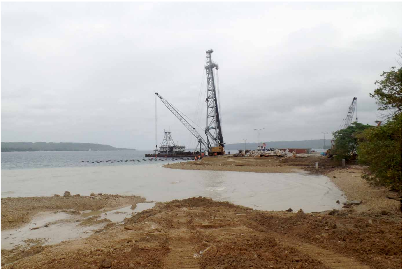
Soil erosion and sediment control measures are important for developments that involve land-moving and earthworks. If these measures are not effectively applied, adjacent waterways can suffer from siltation, which can affect water quality, coral reefs and fish nurseries. Photo: Melanie Bradley
